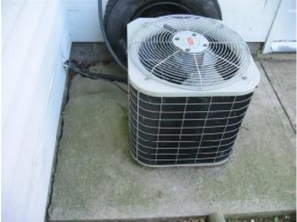
Grounds & Drainage # GD2
