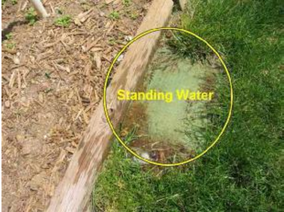
Grounds & Drainage # GD1
