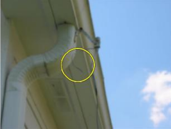
Reattach rain gauge sensor wire
