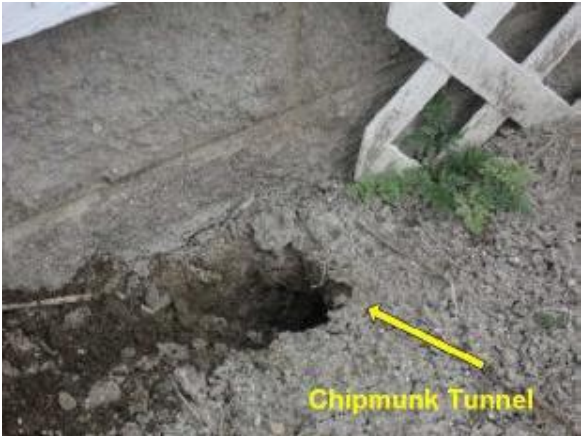
Grounds & Drainage # GD4
